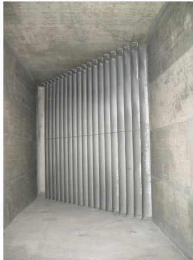
Figure 5: Example of a guide vane, installed in a fresh air duct.
