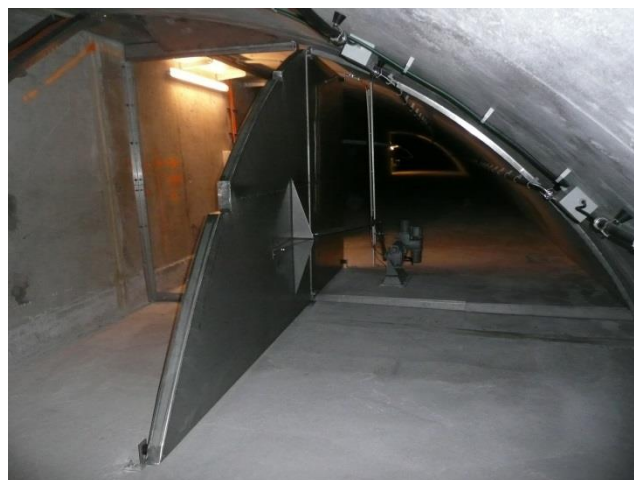
Figure 11: Butterfly flap, which separates the ventilation sections.
